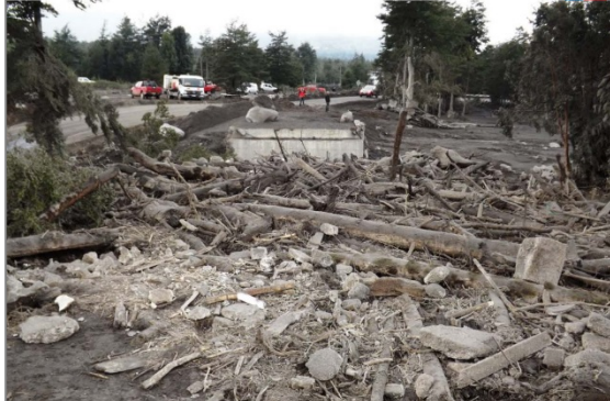
LAHARS DESTROYED BRIDGES
